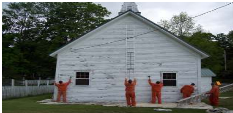
(below) Crew scraping and painting Church in Glenciff
